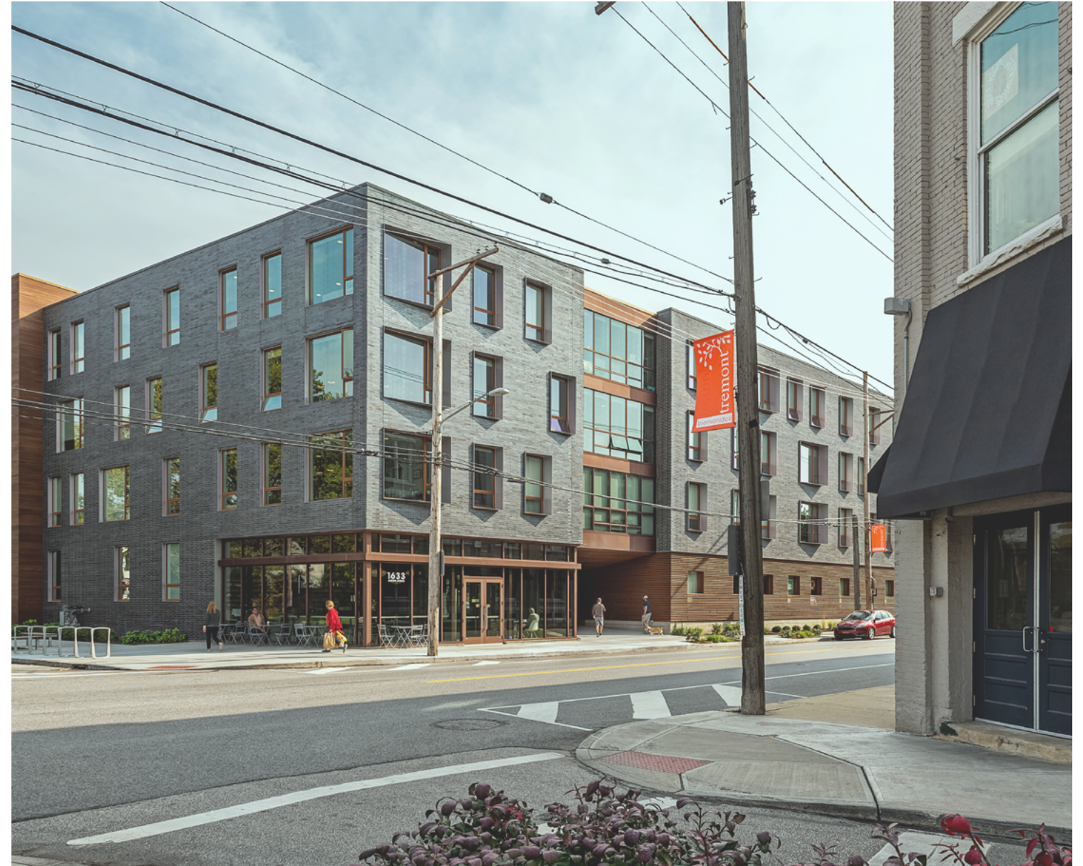
Adjacent Properties - The Tappan + Wagner Awning
