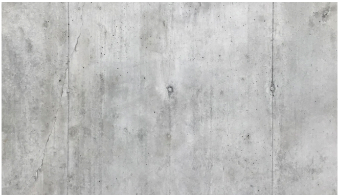
Cast-In-Place Concrete Columns
