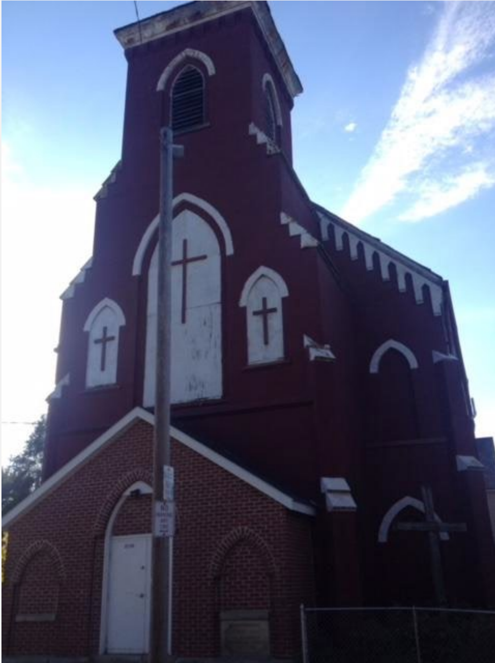
Front views of the church from West 42 nd St.
