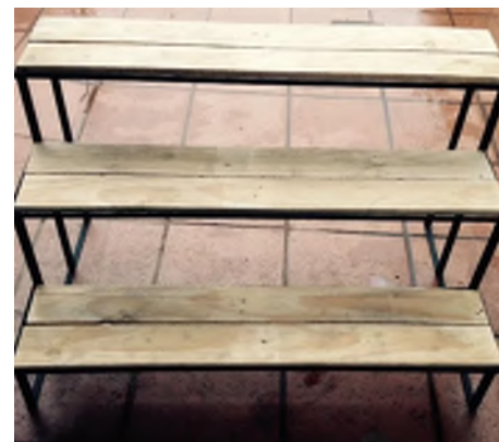
Reference Images - Bleachers Seating Showing Mild Steel Frame and timber bench top.
