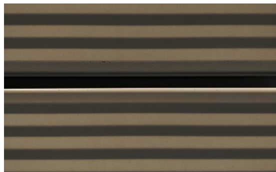
Courtyard - Striated Metal Panels
