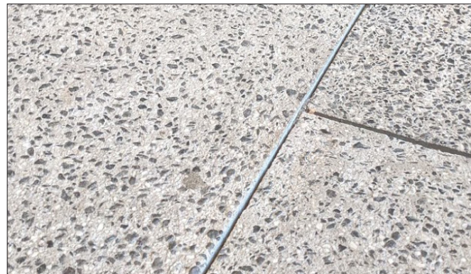
Large Aggregate Concrete
