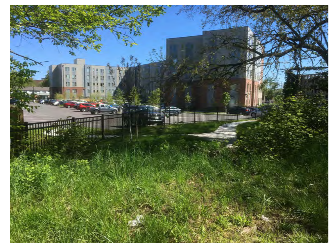
North View - Axis @ Ansel Apartments
