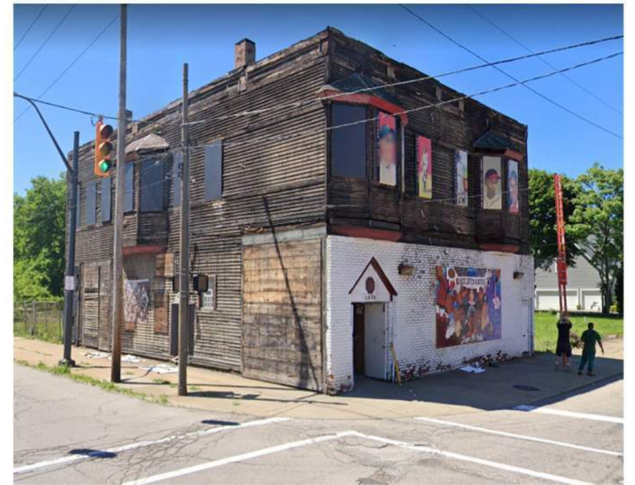
BUILDING NORTHWEST OF INTERSECTION
