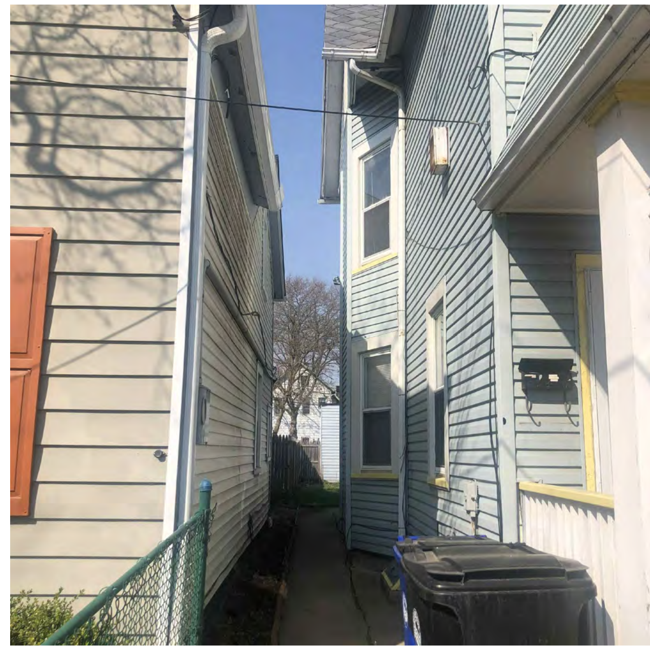
W 44TH STREET - WEST SIDE LESS THAN 3' CLEAR
