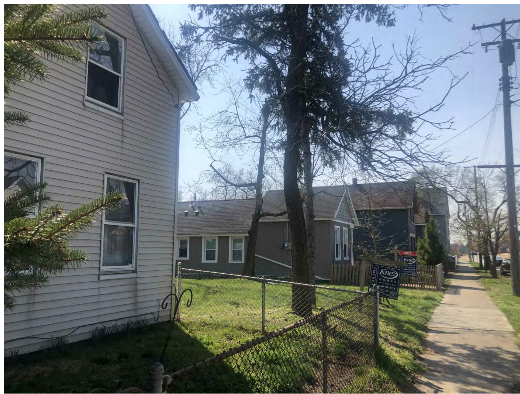
W 44TH STREET FACING SOUTH (SITE FROM SIDEWALK)
