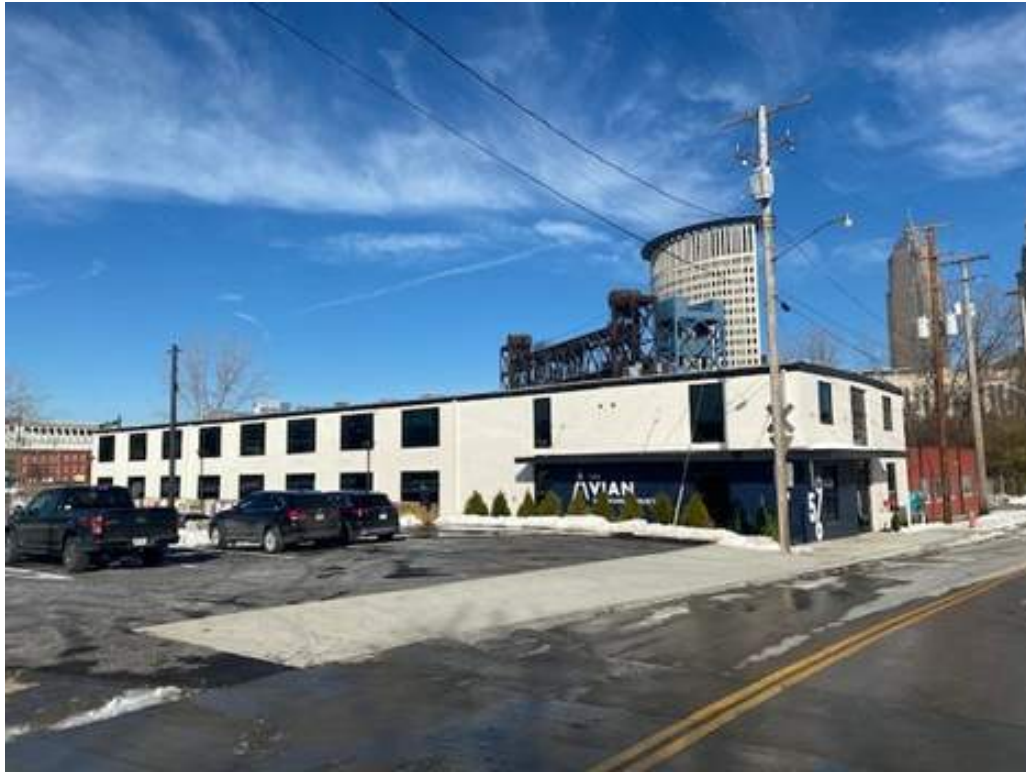
1. FRONT OF BUILDING
