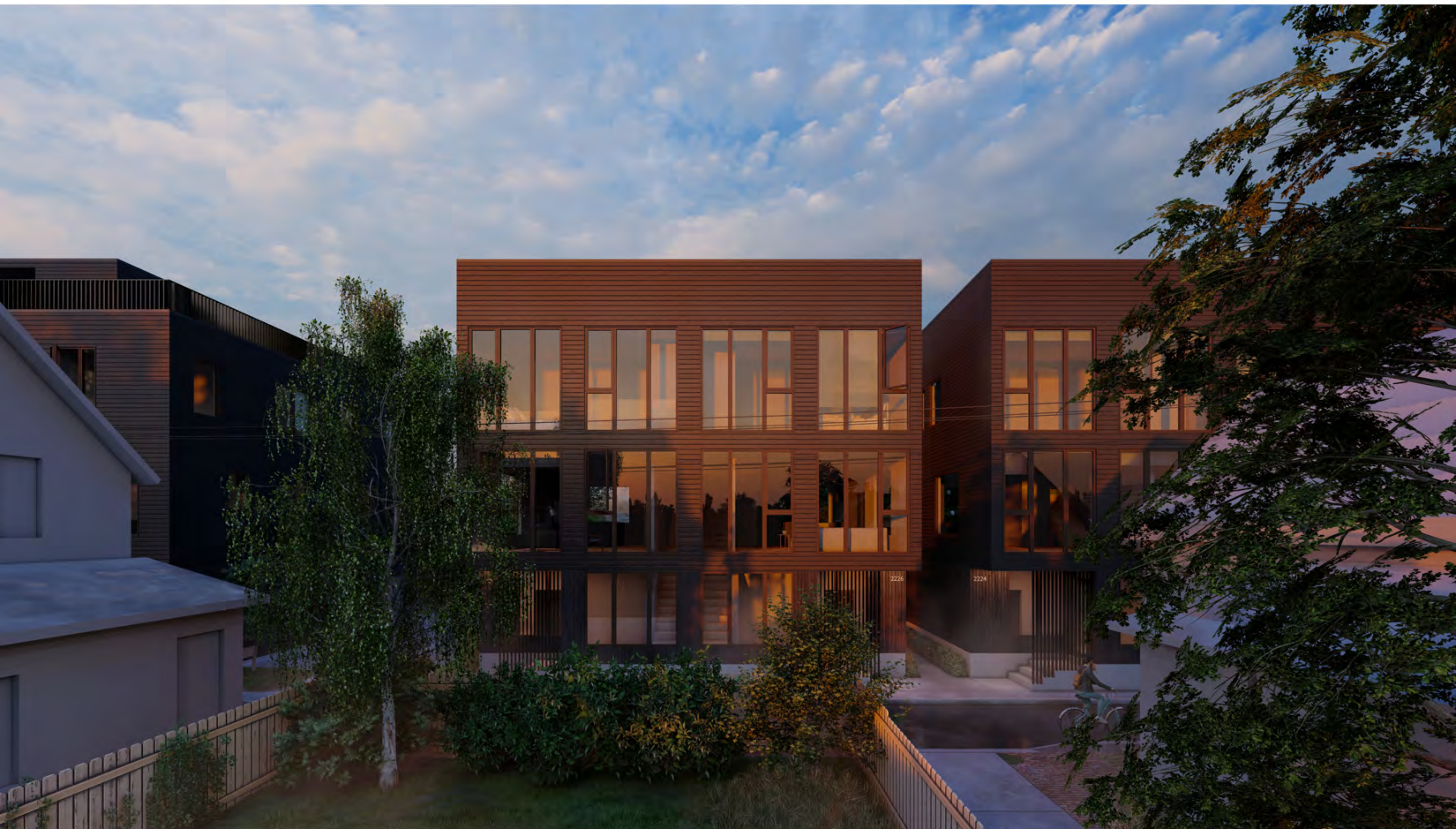
W15th Street Units
