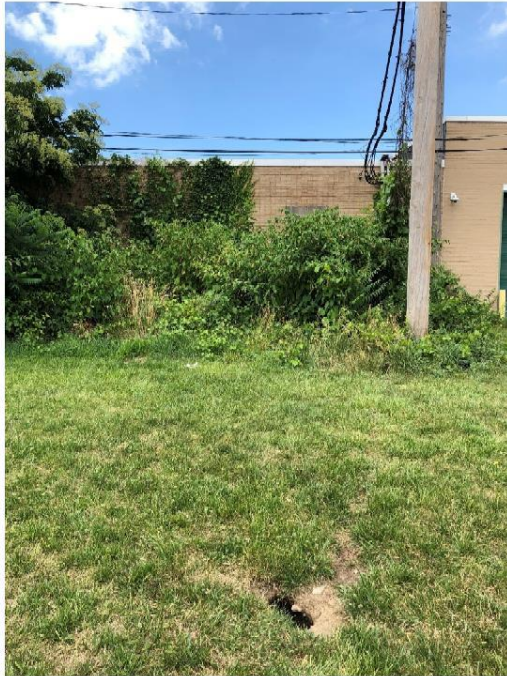
Image 10 – View in more detail of growth on and near existing building. The hole located in the foreground shows remains of an existing foundation. Extent is unknown, but there is potential for this based on site history. See Woodland Parcel Diagram at the end of this narrative about potential existing buried foundations
