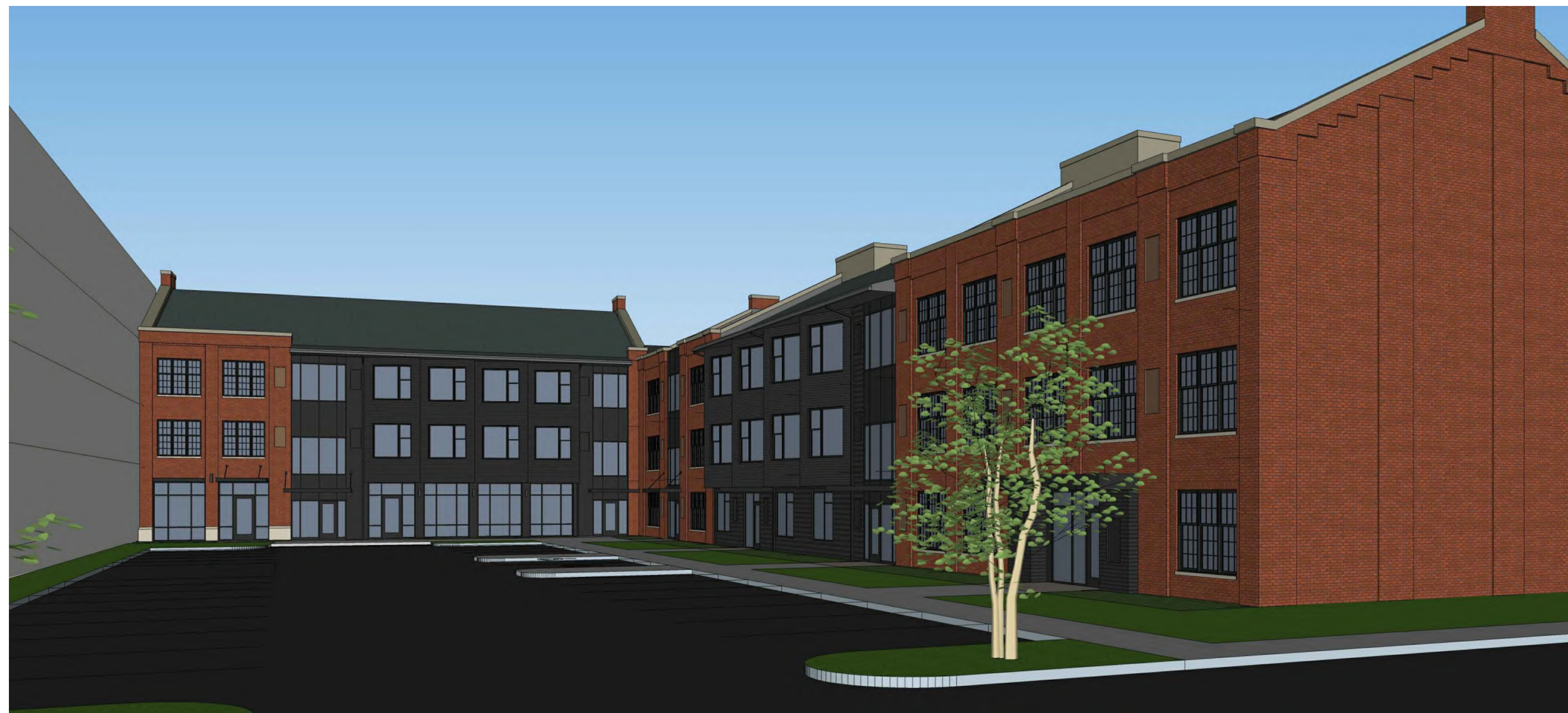
VIEW 8: FROM PARKING BEHIND
