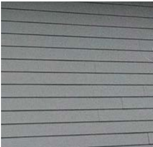
FIBER CEMENT T-1 SIDING AMERICAN FIBER CEMENT COMPANY 030 MERCURY
