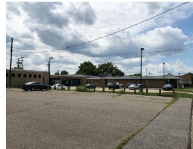
Image 12 – View from Woodland back to existing building. Curb cuts will need to be filled and match with adjacent tree lawn and street curb. Extent of new versus existing to be further evaluated. Sidewalk looks to be in decent condition; a more formal assessment will be needed as to required patching, repairing or full replacement as it relates to the streetscape, new plaza and entry sequence.
