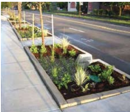
Sidewalk planting to manage stormwater runoff
