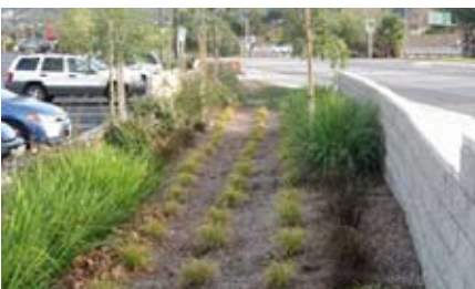
Berms and landscaping with short retaining walls
