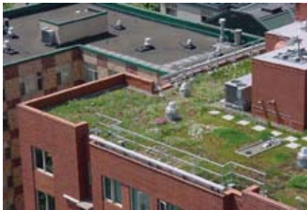
Green roofs help regulate indoor temperatures and onsite management of stormwater
