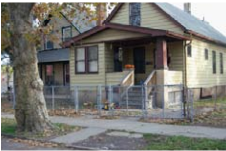
Partly enclosed porch on a historic house
