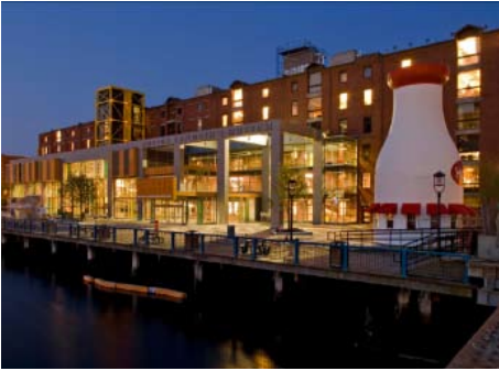
Industrial building reuse
