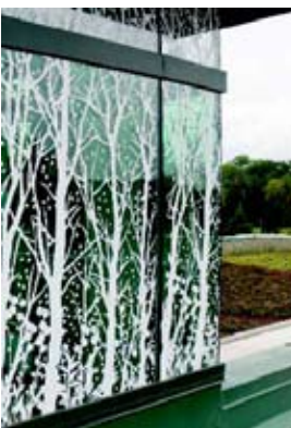
Patterned glass as visual markers to prevent bird 'collisions'
