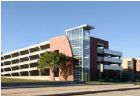
Use of glass for stair and elevator core for the parking facility at Cleveland State University
