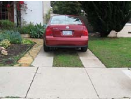
Driveway with partial paving to minimize impervious surface
