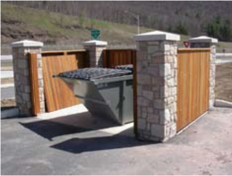
Dumpster enclosure for multi-family residential
