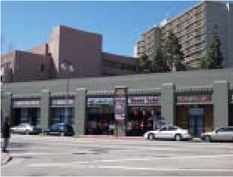
Example of multi-tenant signage
