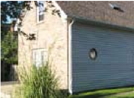
Houses originally made of wood siding must not be replaced with brick
