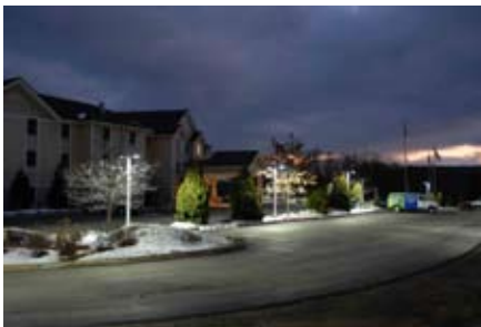
Downward lighting with energy efficient LED bulbs
