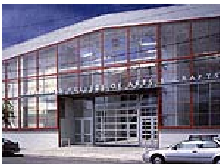
Warehouse converted into art school
