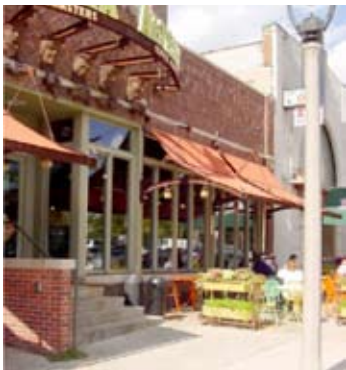
Welcoming entry and overhead weather protection
