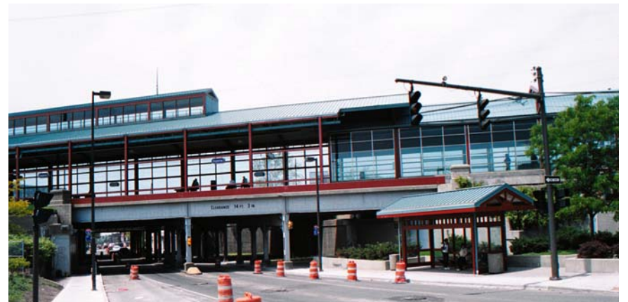
Approaching the Superior Avenue Railroad Bridge from Euclid Avenue
