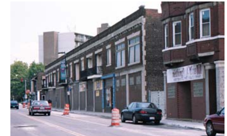
Existing boarded up street edge
