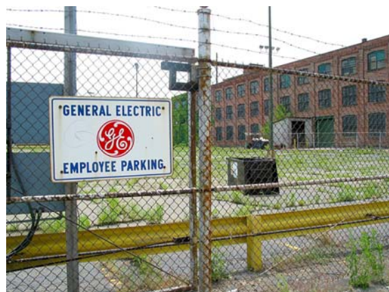
Vacant industrial buildings scattered throughout the city are in need of clean-up and re-use to improve neighborhood image, and environmental and public health. [Former GE Plant – Goodrich-Kirtland Park neighborhood]
