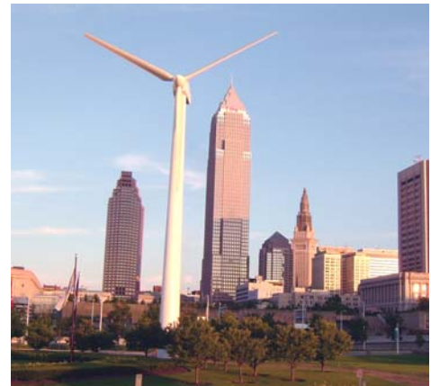
Cleveland’s high profile icon of sustainability. [The Great Lakes Science Center’s Wind Turbine, Downtown]
