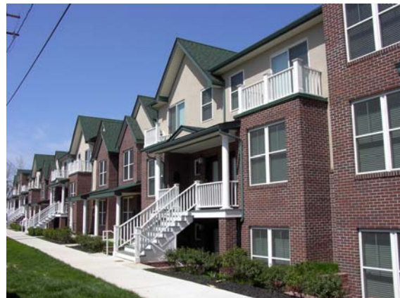
Cleveland’s first infill townhouse project built using green building principles. [Cleveland EcoVillage Townhomes, Detroit-Shoreway neighborhood]
